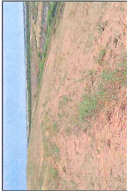
PHOTO 19 Cell vegetated with intermediate cover
