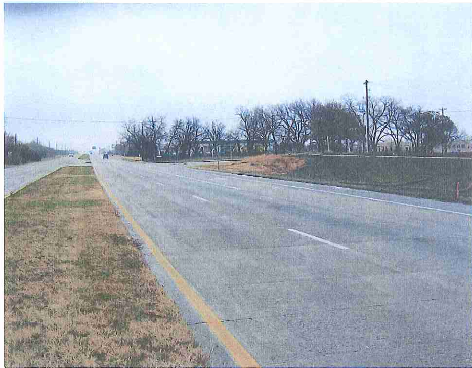
EASTBOUND S.H. 121B AT HUFFINES BOULEVARD INTERSECTION
