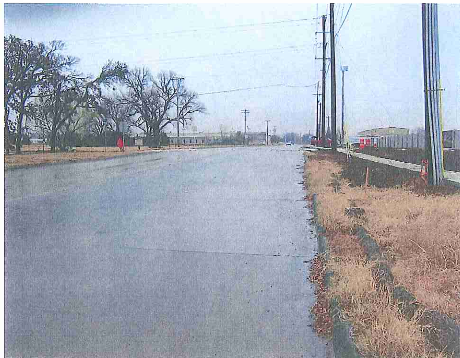
SOUTHBOUND HUFFINES BOULEVARD AT S.H. 121B INTERSECTION
