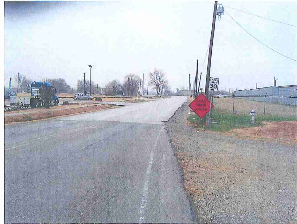
SOUTHBOUND HOLFORDS PRAIRIE ROAD AT S.H. 121B INTERSECTION
